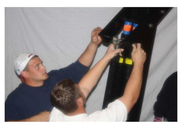
Crank the Lower arm down with the crank and attach the upper extension arms using the 16mm x 10" Bolt and Nut
