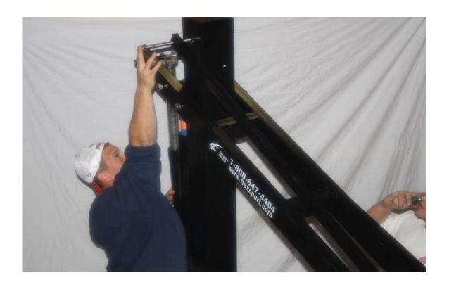
Attach the backboard by raising it up and use a 16mm x 11" bolt to attach the lower extension arm to the lower connection point on the H Bracket
