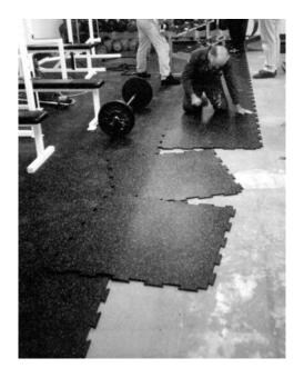
Four-Side Interlock Loose Lay Installation
