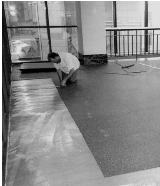
Square Cut Glue Down Installation
